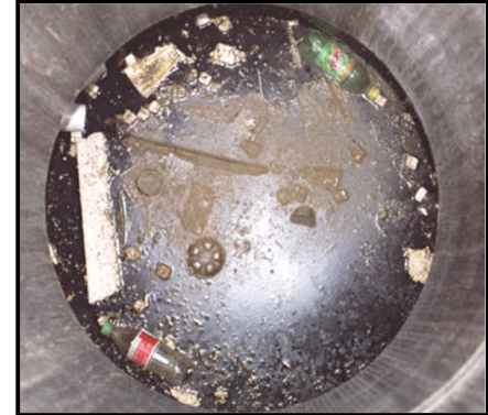
Floatable debris in the AquaSwirl
