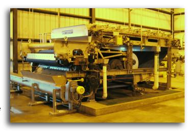
The project team designed the system so pre-screening, additional chemical pretreatment, and pH control can be added later. The entire system, from lift station pump to dewatered solids conveyor, is automatically controlled via a programmable logic controller (PLC) and an Allen-Bradley touch-screen terminal.
