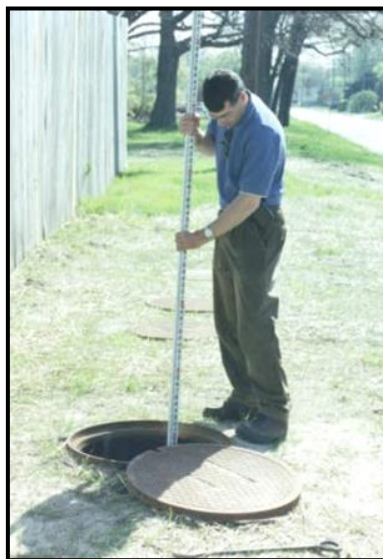
Sediment inspection using a stadia rod
