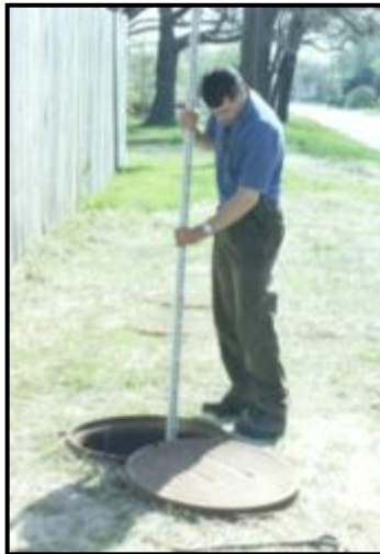
Sediment inspection using a stadia rod in a single chamber.
