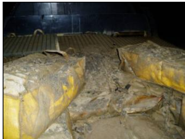
Figure 2. Perlite filter media needs replacement.
